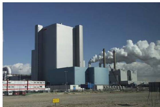
E.On power plant Maasvlakte 3 under construction (Photo: Gualtiero Böhm)
